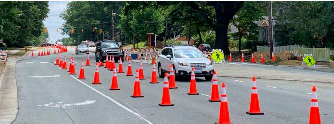
The Durham team constructed a protected pedestrian refuge within the existing median. They also closed a lane of traffic and created a separate space for buses to pull over at the bus stop.
