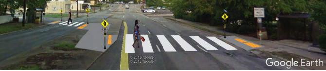
The most common crossing patterns observed at the site were D and C, where no crosswalk was present. Based on these observations, and based on feedback from the community, the Durham team developed a concept to install a new mid-block crosswalk with a protected pedestrian refuge.
