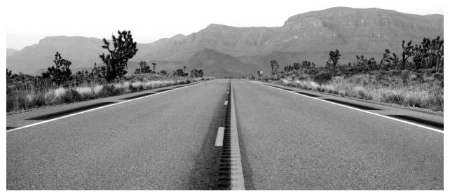
Figure 9. Center and edge line rumble strips on rural roads can be an effective Safe System application to reduce rural road departure fatal crashes. Source: Jesse Collins/Unsplash.
